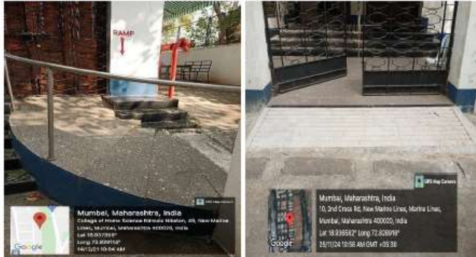
Ramp for wheelchair
