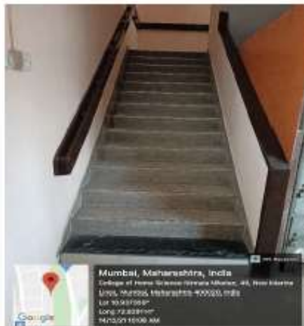
Railing on staircases
