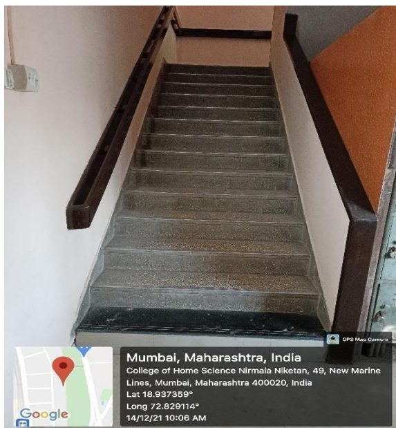
Railing on staircases
