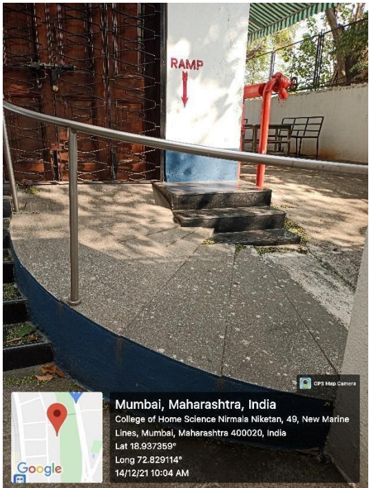
Ramp for wheelchair
