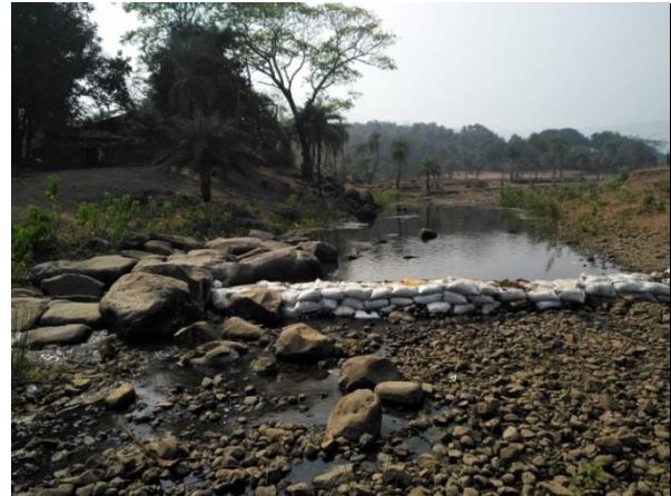
Completed top view of bandhara
