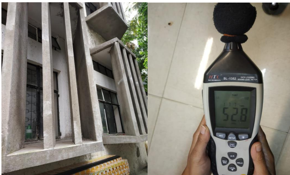
Photo 31: The noise barriers and noise sampling equipment
